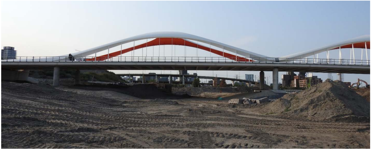
Photo 2 Standing in the river bed, looking north at the new Commissioners Street bridge
